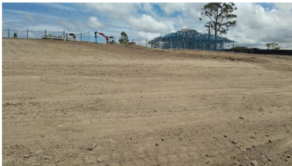
Photograph 13: From north-eastern corner of Lot 719, facing southwest.
