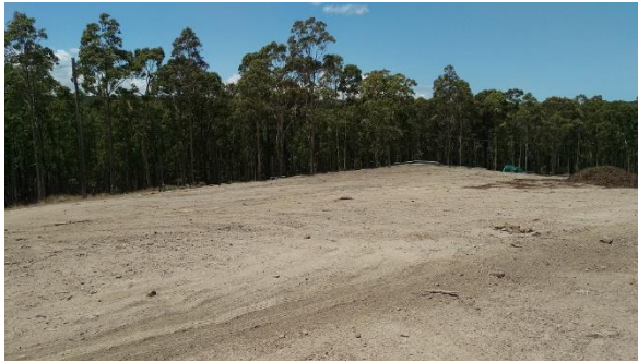
Photograph 9: From south-eastern corner of Lot 719, facing northeast.
