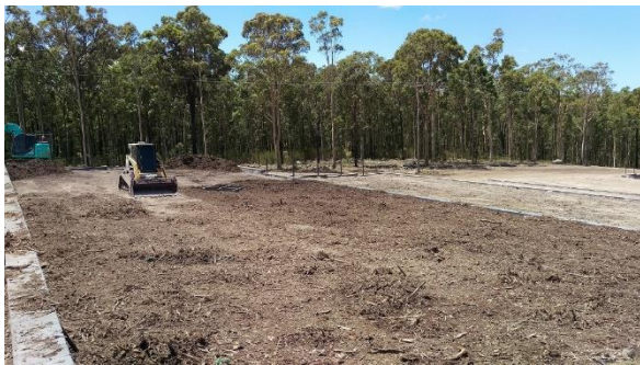
Photograph 5: From south-eastern corner of Lot 713, facing northeast.
