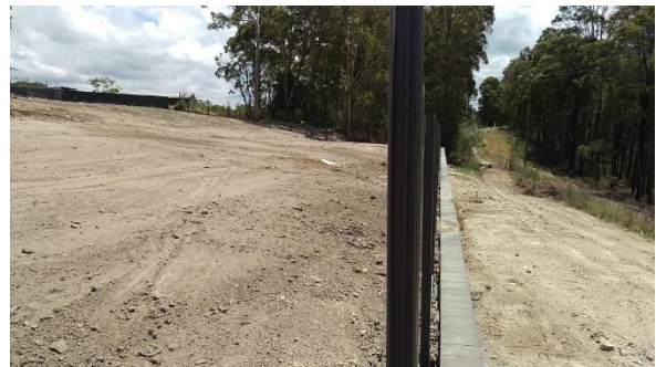
Photograph 14: From north-eastern corner of Lot 719, facing west.
