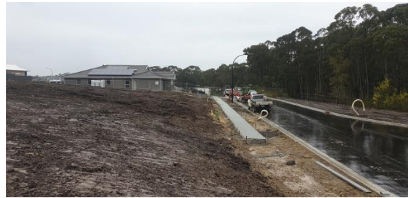
Photograph 2: From near north-western corner of Lot 617, facing south.
