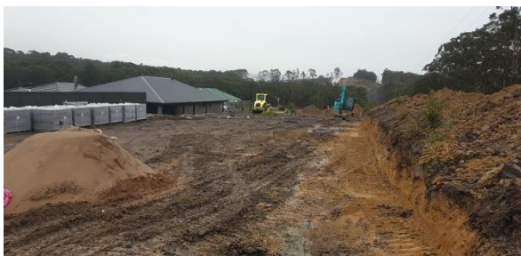
Photograph 7: From north-eastern corner of Lot 625, facing west.
