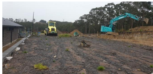
Photograph 6: From eastern boundary of Lot 624, facing west.
