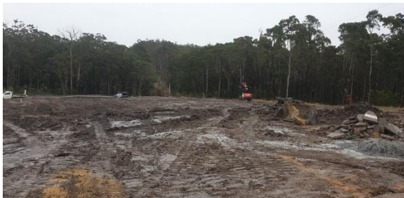
Photograph 3: From near shared boundary of Lots 620 and 621, facing west.
