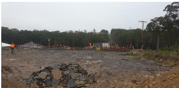
Photograph 5: From eastern boundary of Lot 623, facing west.
