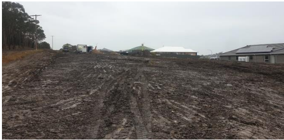
Photograph 1: From near north-western corner of Lot 617, facing southeast.
