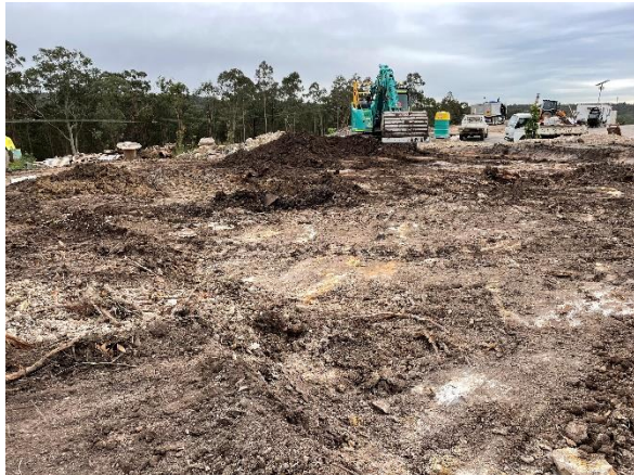
Photograph 15: From near centre of Lot 430, facing east, following removal of additional unsuitable material to underlying residual clay / weathered rock material. Photograph taken on 03/06/22.
