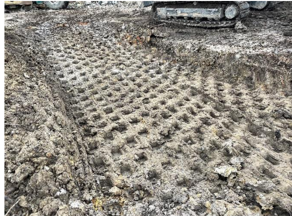
Photograph 16: From near north-western corner of Lot 430, showing placement and compaction of backfilled area under level 1 supervision. Photograph taken on 03/06/22.
