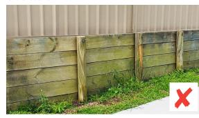
**RETAINING WALLS** – timber retaining walls that are visible from a public place are discouraged.
